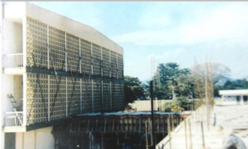
Block C under construction
