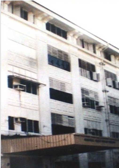
Block A, Penang General Hospital, 1949
