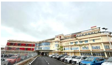
Image 18 Hospital Tawau Sabah
