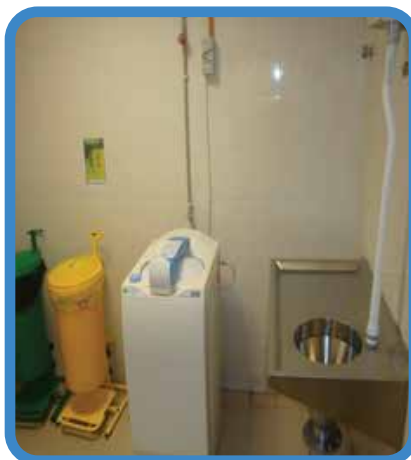
Dirty Utility Room
