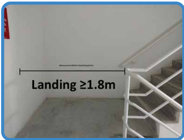
Measurement is from wall to handrail
