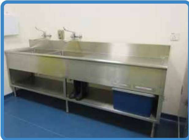
Dirty Utility Room
