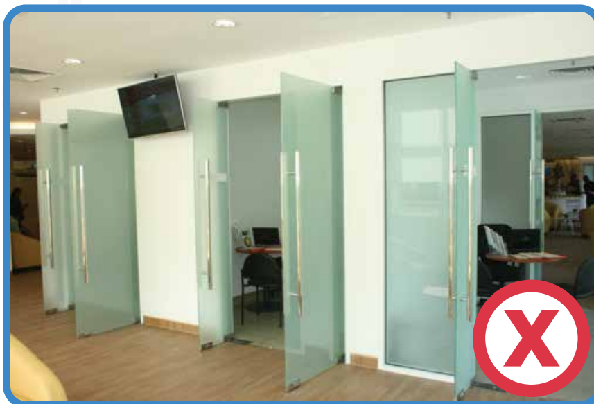
Doors should not swing into corridors
